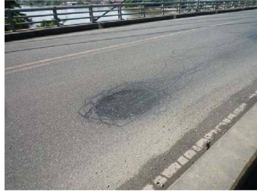
Pothole on the bridge carriageway (repaired)
