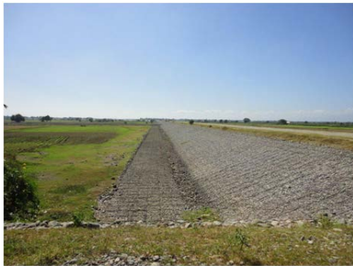
Closure Dike (taken from side)
