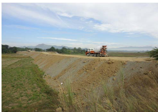
Earth dike extension work (using local fund)
