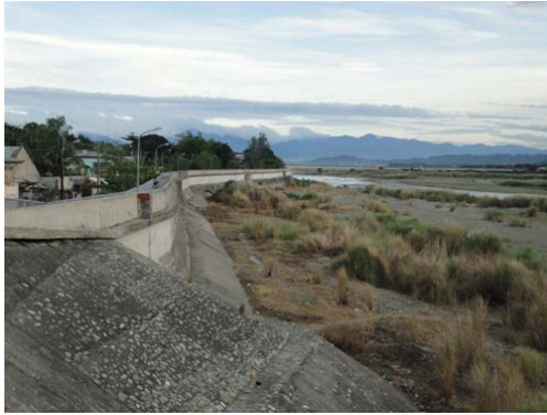
Riverwall in Laoag City
