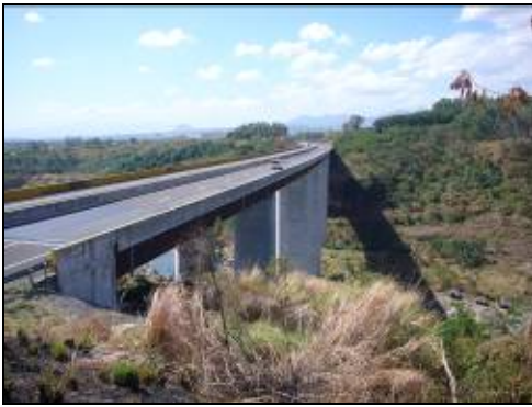
Gumain River Bridge
