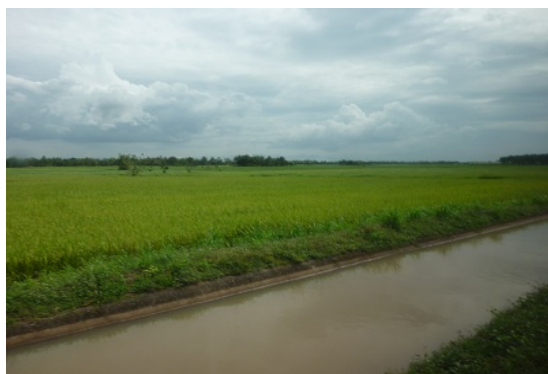
Figure 13: Rehabilitated Main Canal
