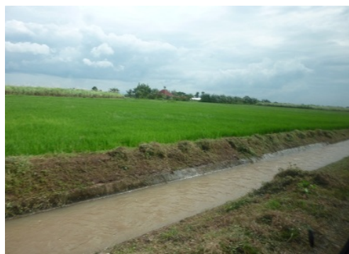
Rehabilitated Secondary Canal
