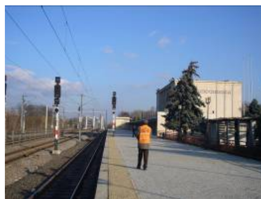
Ending point of Bucharest North - Baneasa section (Baneasa Station)
