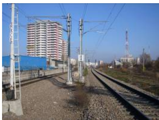
Beginning point of Bucharest - Baneasa section (Bucharest Station)
