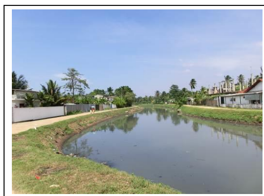
Drainage constructed by the project
