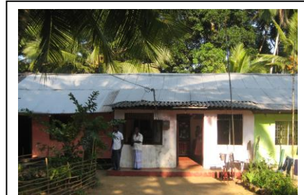
Figure 2: Reroofed Line Room
