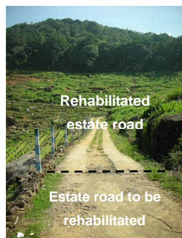
Figure 5: Rehabilitation of Estate Roads
