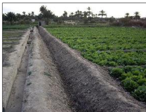
Concrete canal and old canal (Gabs)
