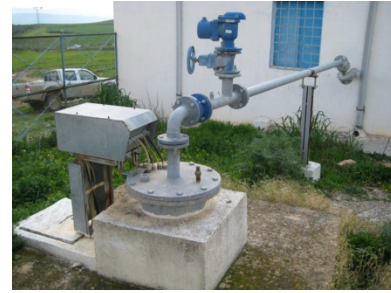
Pumping Facility (Gmara Village, Beja Governorate)
