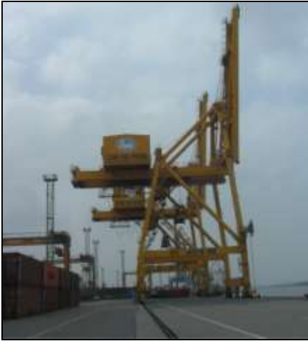
Cranes procured in the Project
