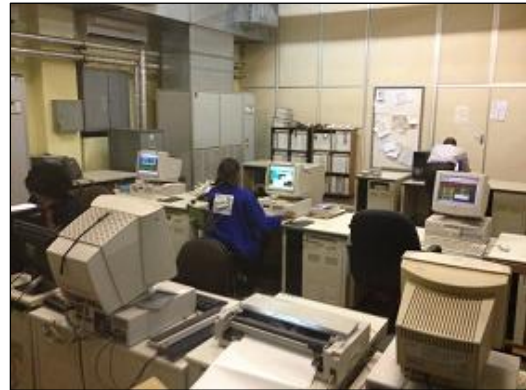
Central Management and Operations Center (Bulawayo)
