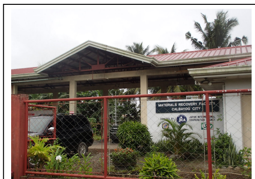
Material Recovery Facility (Calbayog City)
