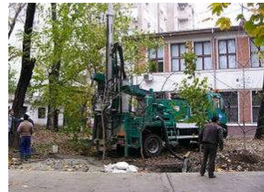
Survey on the conditions of soil and ground
