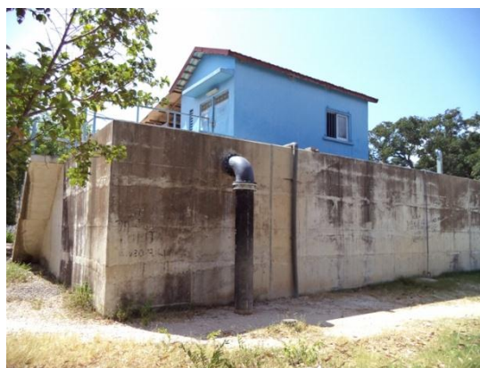
Welezo Reservoir developed in the project
