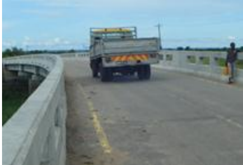
Replaced bridge (Cuacua I)
