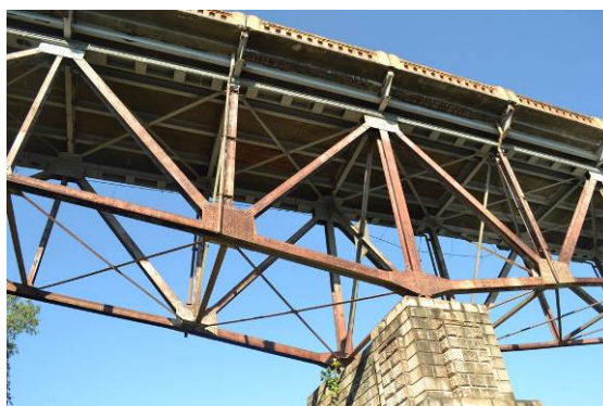
Truss member (rusted) and concrete slab (exposed reinforcing bars) of the Old Bridge
