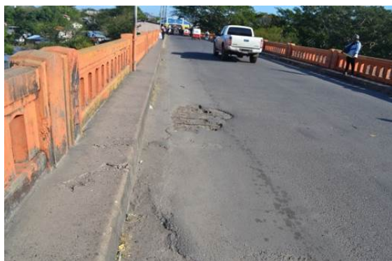
Damaged road surface of the Old Bridge
