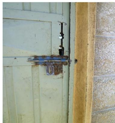
Figure 2 Broken door knob & key hole that is changed to a bar key
