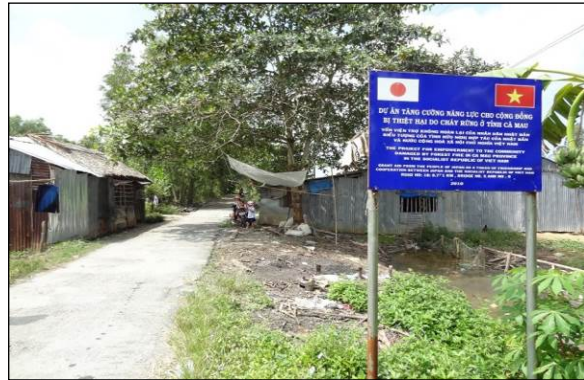
Constructed road (Ngyen Phich Commune, U Minh District)
