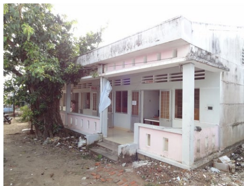
Photo 4: Building of a health station (Khanh Binh Tay Bac)
