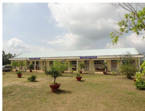
Photo 3: Constructed primary school building (Lam Ngu Truong I Primary School)
