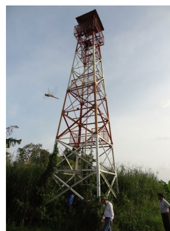
Photo 2: Constructed Forest fire monitoring tower (U Minh Ha National Park).
