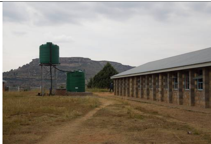
The classroom and water tower of the school in Leribe district
