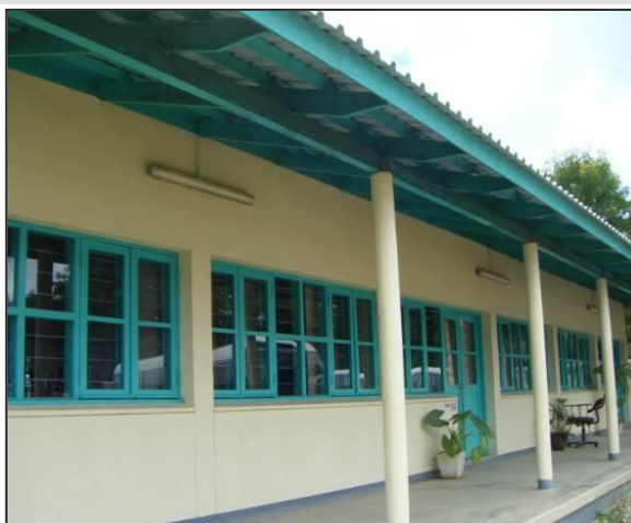
Constructed classroom (CFS Massinga)
