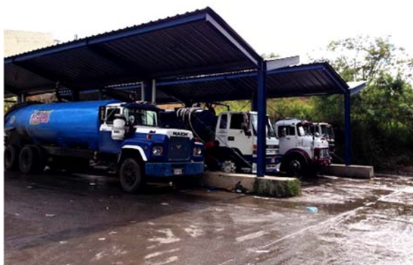
Laureles Water Filling Station
