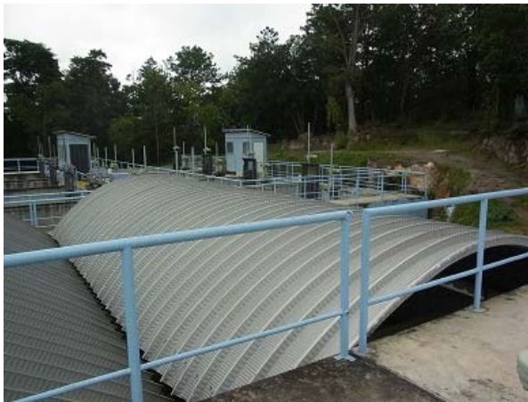
Settling basin and filter basin added to the Picacho WTP
