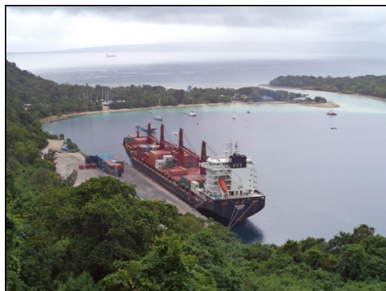
Main Wharf rehabilitated in this project and a cargo ship calling at the port
