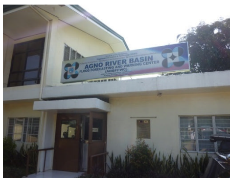
Rehabilitated Agno Sub Center
