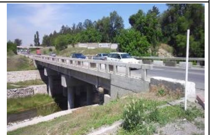
The Alamedin Bridge
