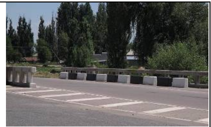
Painted and repaired shoulder in the Ken-Bulun bridge
