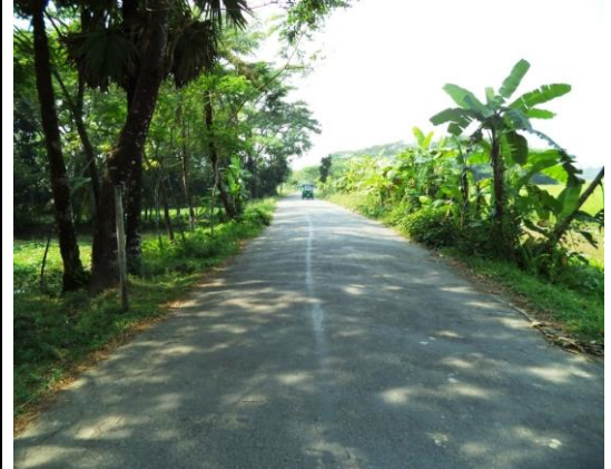
An improved road in Noakhali District
