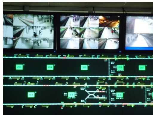
Remote Control and Surveillance System
