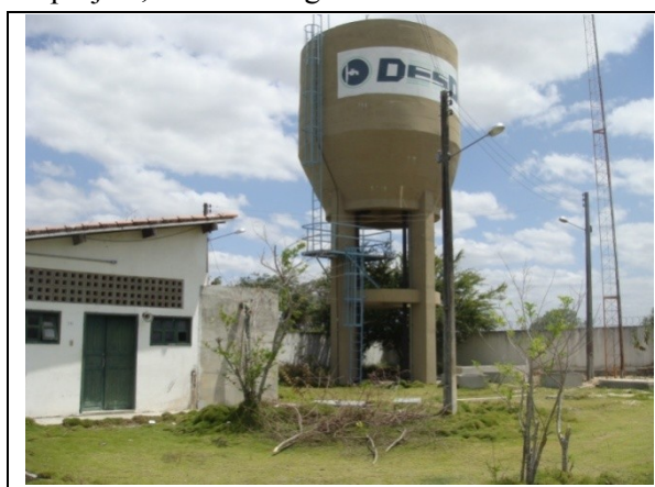
Figure 6: A Water Supply Tank for the Alto Sertão Water Conveyance System
