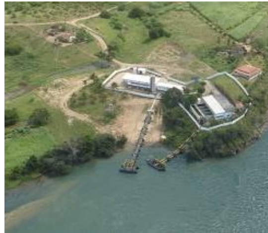
An intake and purification plant for a Semi-Arid water supply system
