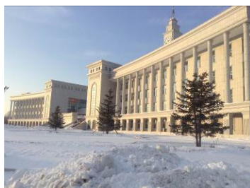
Part of this building was constructed as an additional output of this project. A common laboratory (equipment sharing platform) was established there.
