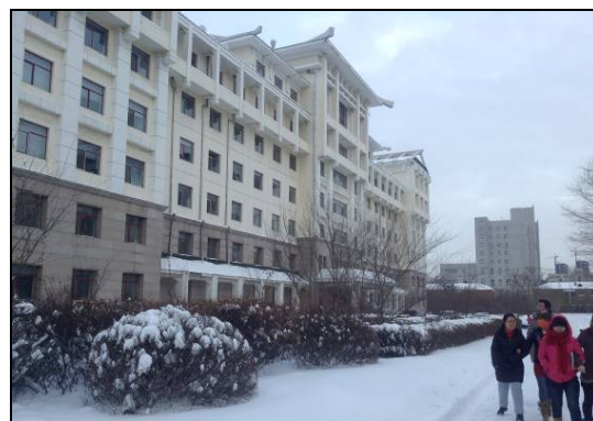
Building of the School of Pharmacy (Harbin Medical University)
