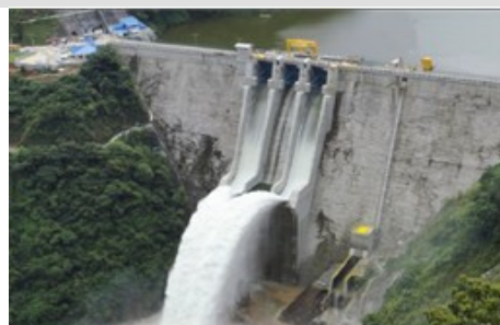
Pirris Hydroelectric Power Plant RCC 2 Dam (provided by Costa Rican Institute of Electricity, ICE)
