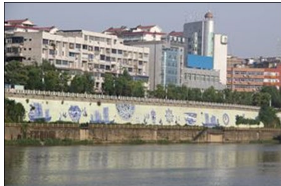
In Jingdezhen city, dikes have been constructed or repaired featuring the culture of ceramics and protection of the ecosystem.
