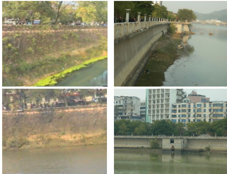
Photo 1: Shibeidike at Shangrao city The photos on the left show conditions before the Project while the photos on the right show conditions after.
