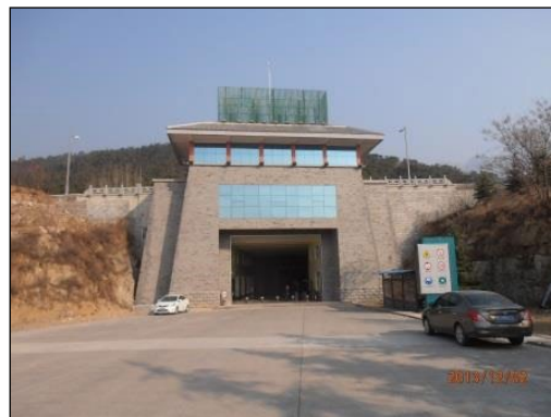
Entrance of Underground Power Station
