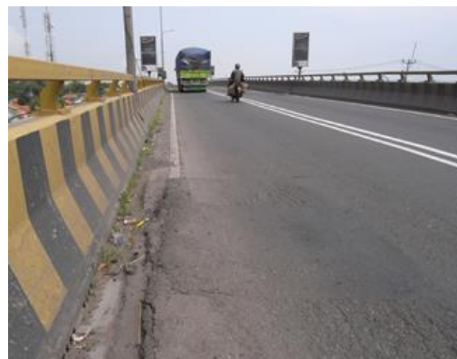
Photo6. Patch repair and drainage ditch. The lid of the ditch cannot be opened (Geban FO)
