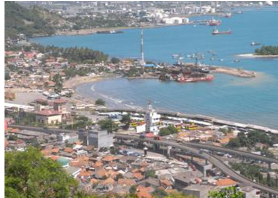
A distant view of Merak flyover
