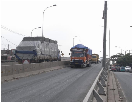
Photo 1. Trucks with heavy loads passing over the flyover (Balaraja FO)
