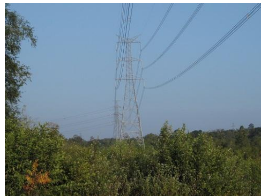
Transmission lines constructed under the project
