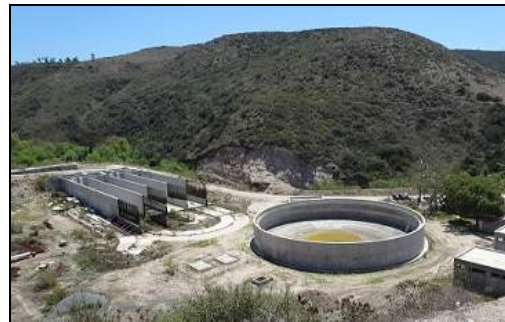
Figure 5: The Unfinished Tecolote-La Gloria Sewage Treatment Plant (at the time of the Ex-Post Evaluation)
