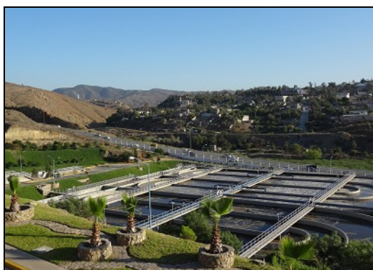
Monte de Los Olivos Sewage Treatment Plant (Tijuana)
