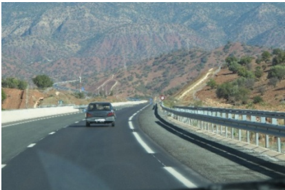
Motorway constructed under the project (the Argana to Ameskroud segment financed by the project)
