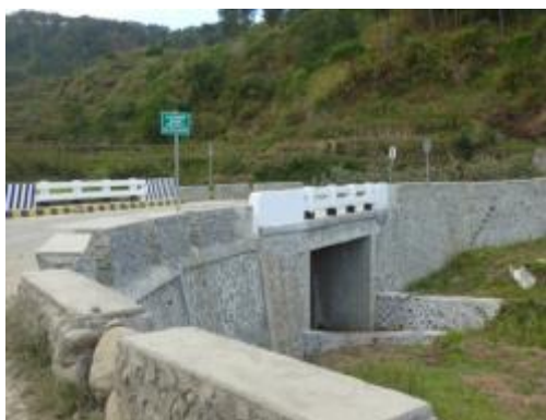
Photo 3: Bridge Developed by The project
