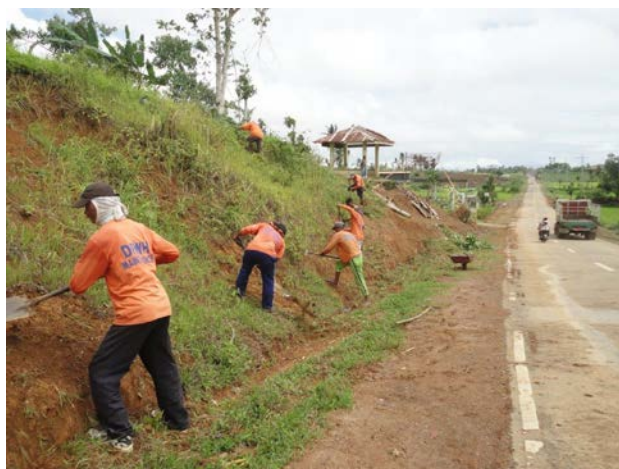
Road Maintenance Crew
