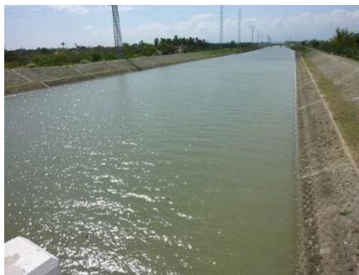
Jaro Floodway Constructed by the Project
