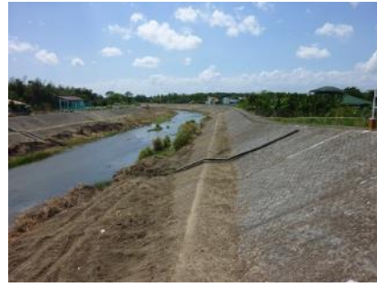
Photo 2: Tigum River after the River Improvement Works
