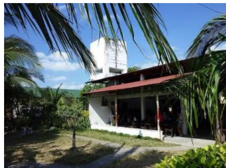
Photo 4: Facilities Developed in So-oc (From front: church and water tower)
