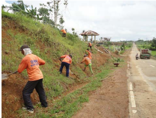
Road Maintenance Crew
