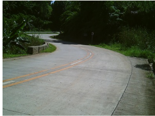
Winding roads in the mountainous area (Section 2 )
