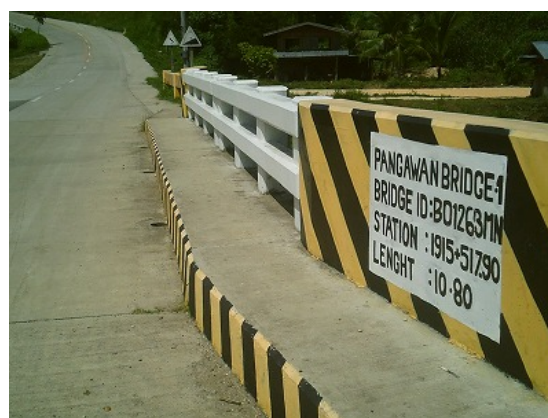
Rehabilitated Bridge 1, Section 3
