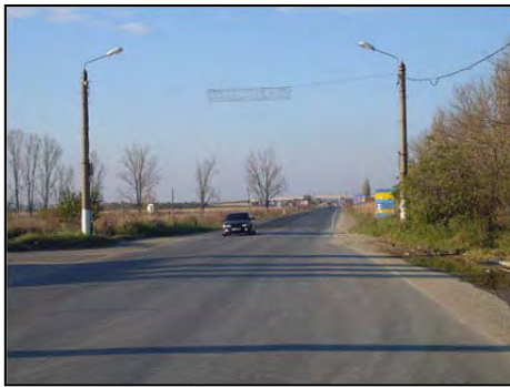
Ending point of Timisoara - Lugoj Road (2-lane section)
