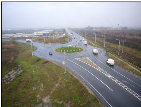
Ending Point of Craiova Bypass
