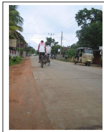
Road reconstructed by the Project
