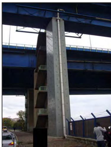
New Golden Horn Bridge Reinforcement of piers (bound with steel plate)
