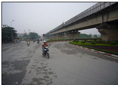
Thang Long Bridge South - Dike Road
