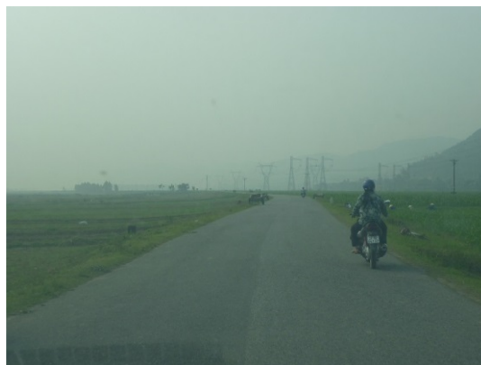
Rehabilitated National Road 15A
