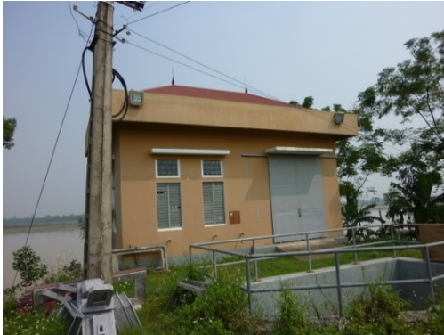
Photo 1: Rehabilitated Nam Trung Pumping Station
