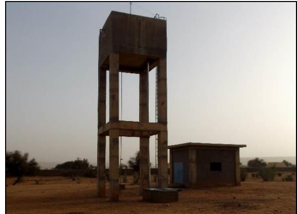
Water Supply Facility Constructed by the Project
