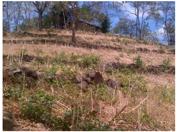
(Stone-lined soil prevention works in El Sauce)
