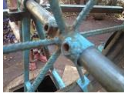
Photo. 5. The wheel of a rope pump that is not working because it has had its bolt removed (Bolosore Woreda, Wolayita Zone) (Photo by the evaluator)
