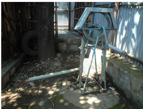
Household rope pump installed in the Project 2
