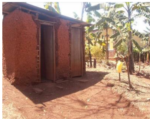
Toilet with hand washing station
